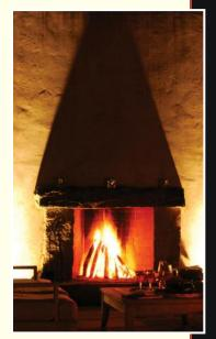
wood more efficiently. This was in part thanks to the restriction in their chimney openings, which helps increase the up draft & allows heat and light to radiate outwards. Today, Rumford fireplaces are enjoying a comeback.
