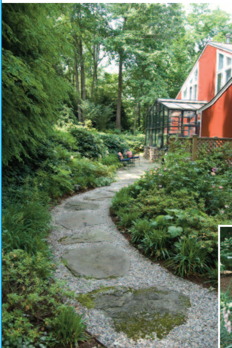
As the homeowner ages, Hoffman's maintenance crew is asked to go the extra mile by providing upgrades around the property. Walkways were made more easily passable and sure-footed by resetting the original natural stone pavers in wider, level courses of small stone to provide confident footing. Masonry seating areas of large stones or dry-work seating walls were also added.
